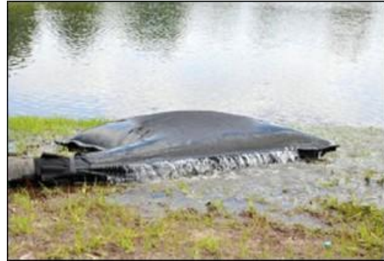
Plate 2-2 Silt bag under inspection
